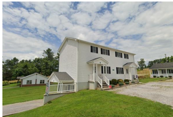
Ron Hughes Apartments
