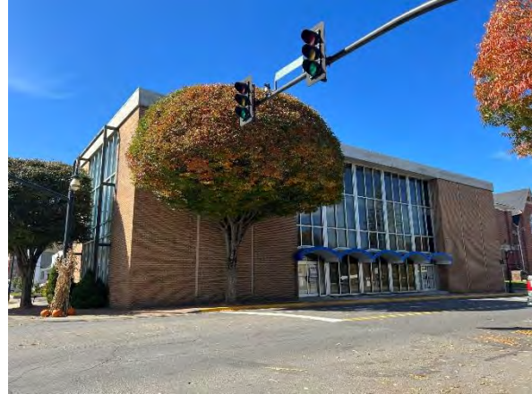
Former Bank Building
