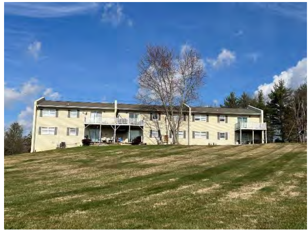
Mountain Empire Apartments
