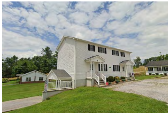
Ron Hughes Apartments
