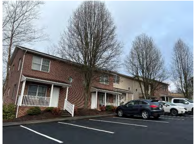
Wyndale Court Condominiums
